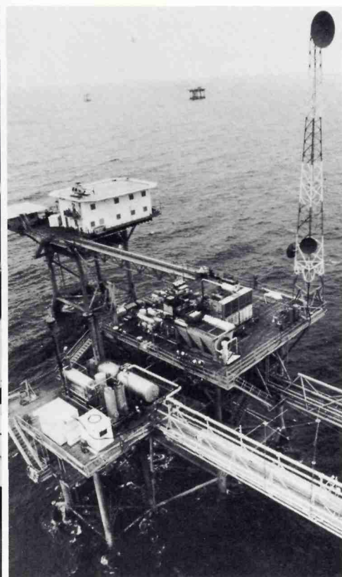
Better management coordination can be achieved with Motorola microwave systems which provide a fixed-path communications network for the petroleum industry. The system carries radio, closed-circuit television, data and several other forms of communication.
