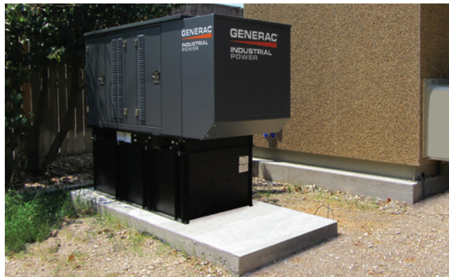
Motorola Alternative Building 10x12 foot with an optional outdoor generator based on the selected equipment load configuration.
