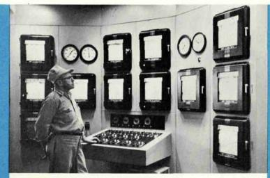
Cross-country meter reader. From one central office, Motorola power line carrier and supervisory control make it possible to meter the flow of gas, electricity, oil or water through lines hundreds of miles away.
