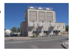
The site connects four impacted water supply wells to a central treatment facility for removal of TCE using air stripping. The wells have a maximum combined extraction rate of around 9,000 gpm and are used to provide treated water to the COS drinking water system. Over the years, the groundwater extraction and treatment rate has decreased to an average of around 3,000 gallons per minute.
