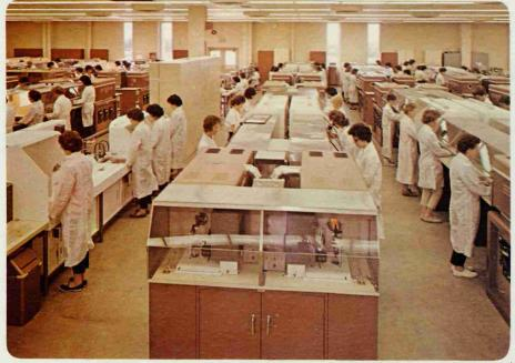
Carefully controlled conditions enable the Division to manufacture integrated circuits to exacting customer specifications. Here are rows of furnaces where various steps, such as diffusion and oxidation, are performed in sequence on integrated circuit wafers. Temperature, pressures and composition of the gases are strictly regulated.
