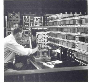
Airborne digital computors undergoing reliability tests above are examples of the "sophisticated hardware" being developed by technical personnel in Motorola's Military Electronics Division.
